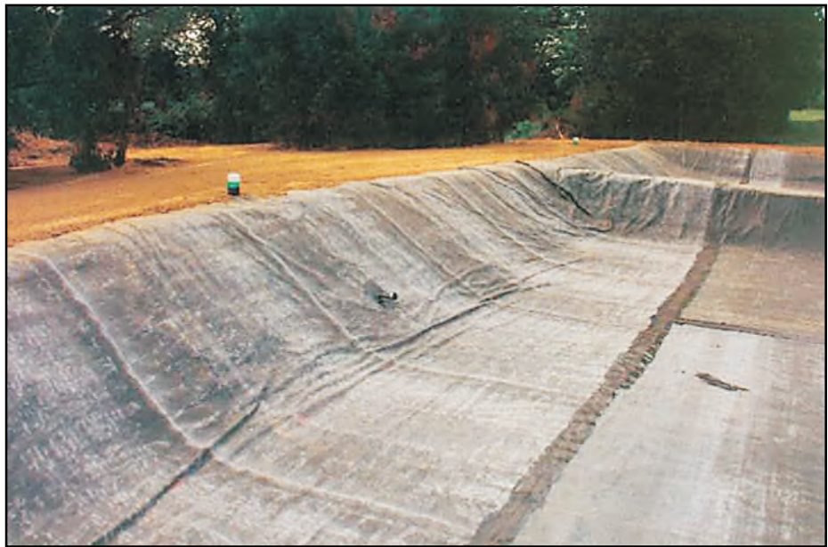
Advantages to using an EPDM rubber liner include conformity to odd shapes and ease of installation.
