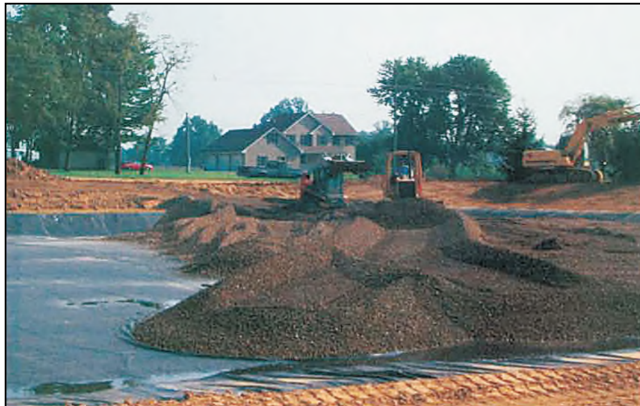
After minimal training from a company representative, Rose Acre Farms was able to install the liner themselves.
