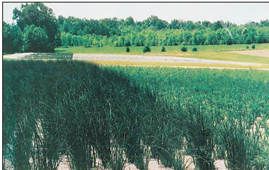
Rose Acre Farms is convinced that constructed wetlands are an environmentally responsible, economical and low maintenance option. Shown above: Photo taken one year after completion.
