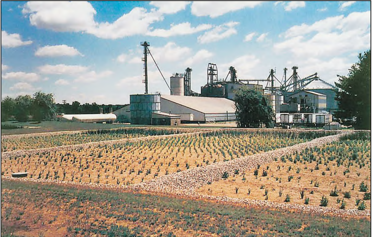
Rose Acre Farms installed both wastewater and storm water constructed wetlands to provide environmentally sound water treatment, while reducing operating and maintenance costs. Shown above: Rose Acre Farms several days after project was completed.
