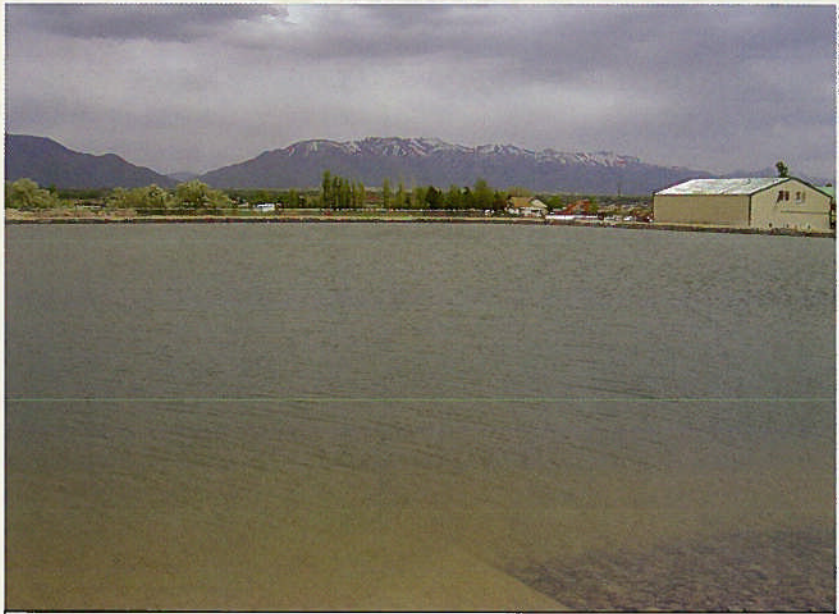
Photo 2. The completed reservoir. Differences in polymeric liner costs (materials and installation) were found to be comparable; hence, an EPDM liner was chosen for what the client and designer saw as a future reparability advantage (after performance needs were met).
