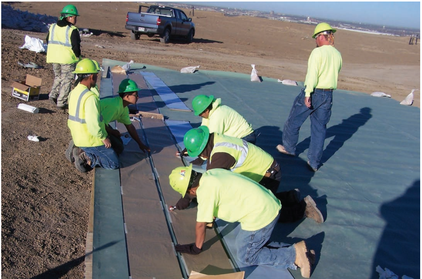
On the Tessman Road Landfill Solar Energy Cover, 1,050 panels were adhered to the exposed geomembrane.
